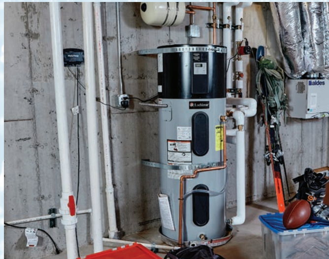
By moving heat instead of creating it, a heat pump water heater uses 60% less energy than electric storage water heaters. PHOTO COURTESY OF HOT WATER SOLUTIONS
