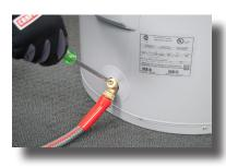
nect) or gas to the tank, then cool its water by opening the hot-water tap on a sink faucet for a few minutes. Close the heater's water supply valve, run a garden hose from the tank's
