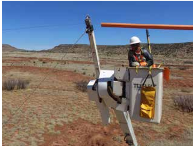
FEC Lineman Phillip Gage doing pole change-out
